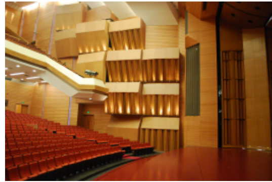
Figure 12. Side wall reflectors in Beijing Television Studio angled to create controlled distribution of early and later sound
