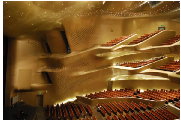
Figure 13. Curved side walls used to generate early reflections in the Guangzhou Opera House
