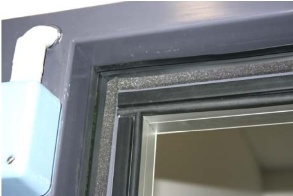
Figure 8. Acoustic rated door showing “batwing”, magnetic and compression seals to head and jamb
