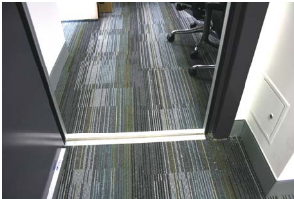
Figure 6. Acoustic rated door showing threshold seal
