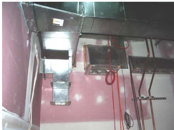
Figure 1. These ducts were extended to provide sufficient attenuation between the Top Secret room and plantroom (photo shows ducts prior to extension)
