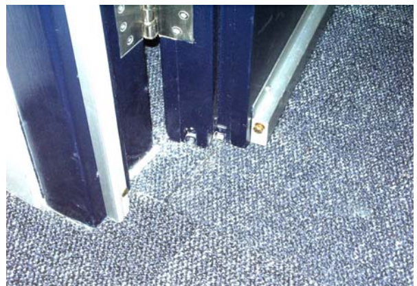
Figure 5. Acoustic rated door seals. Note three drop seals to the base of the door (two fully mortised into the door and one surface mounted) to minimise noise leakage via the threshold.
