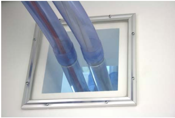
Figure 3. Double glazed vision panel around secret room cables
