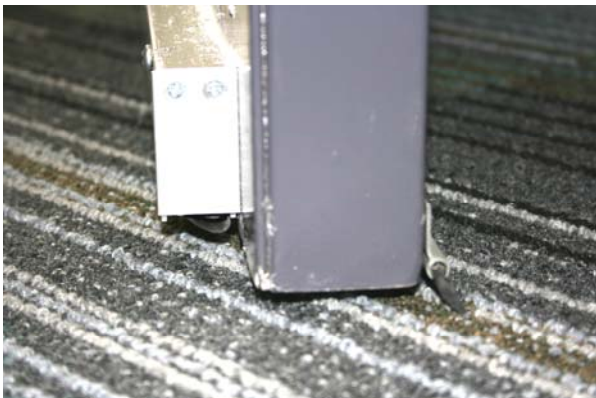
Figure 9. Acoustic rated door showing surface mounted drop seal and sweep seal to base of the door
