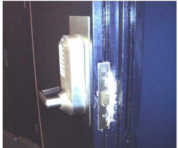
Figure 7. Timber acoustic rated door with seals removed for fitting of door lock
