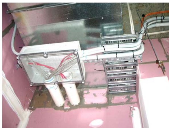
Figure 2. Transparent cable connection boxes. Note sealing around penetrations
