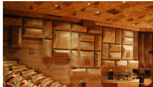
Figure 10. Facets fitted to the side walls at balcony level
