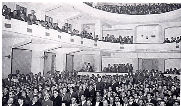
Figure 2. Inside the theatre (about 1965)
