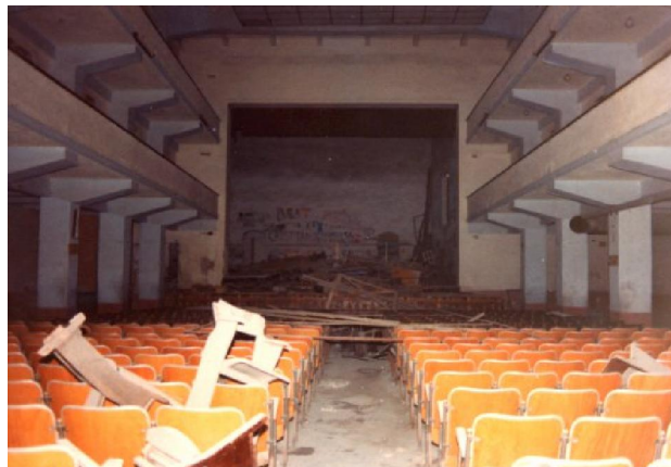
Figure 3. Inside the theatre (after 1982)
