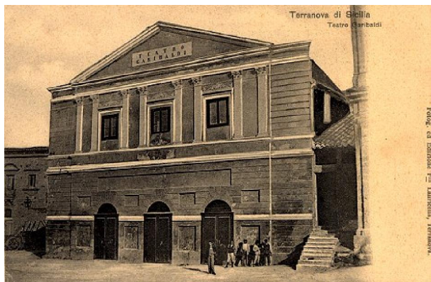
Figure 1. The façade of the Teatro Eschilo at early ‘900
