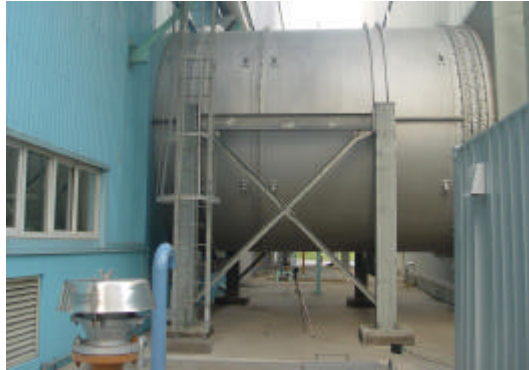
Figure 2. Noise measurement at the exhaust duct of a gas turbine
