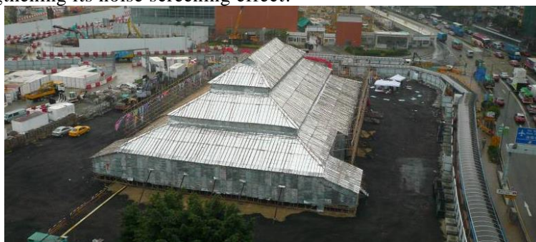
Figure 3 – Bamboo theatre with double layer of metal sheeting
