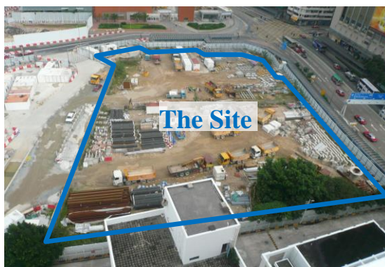
Figure 1 – The temporarily idle construction site
