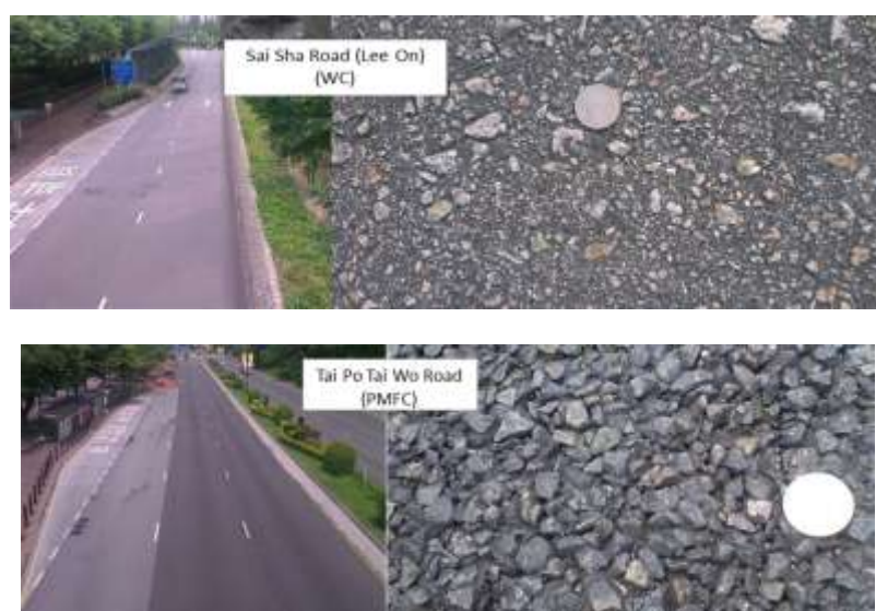
Figure 7: Selected test road surfaces
