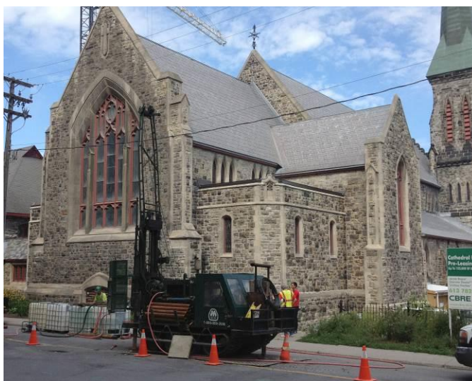
Figure 1 – Borehole Testing at Historic Church
