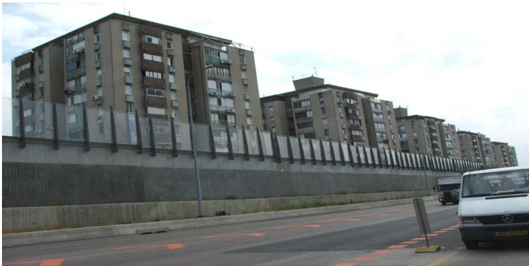
Figure 1 – Typical situation for façade treatment
