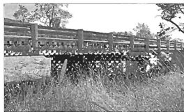
Figure 4 A two span bridge from Cabonne Council in NSW
