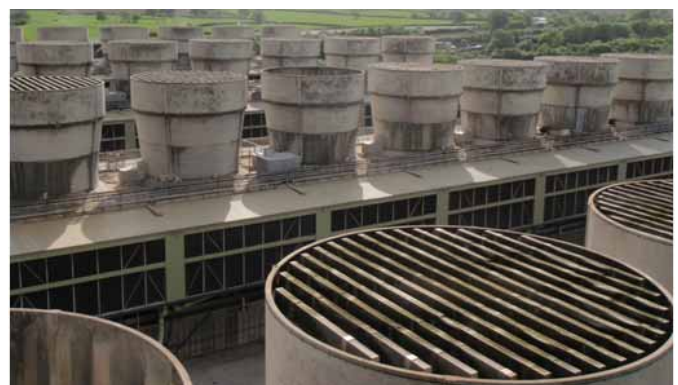
Figure 2. Noise attenuation baffles at fan outlet.
