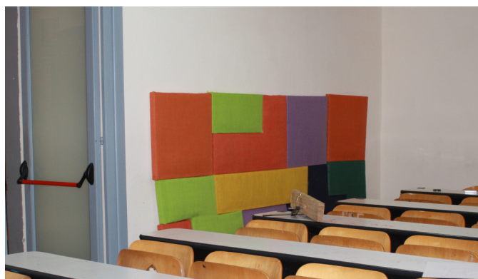
Figure 12. Sound absorbent panels inserted in a classroom
