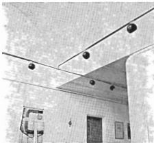
Curved Ripple Sound ceiling in Entrance Foyer
