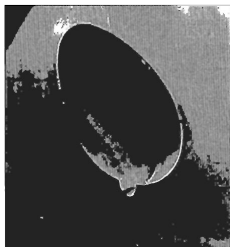
Figure 2. A speaker unit, mounted in the exhaust stack (view from inside the exhaust stack). Note the spout at the bottom to drain any residual liquid after cleaning.
