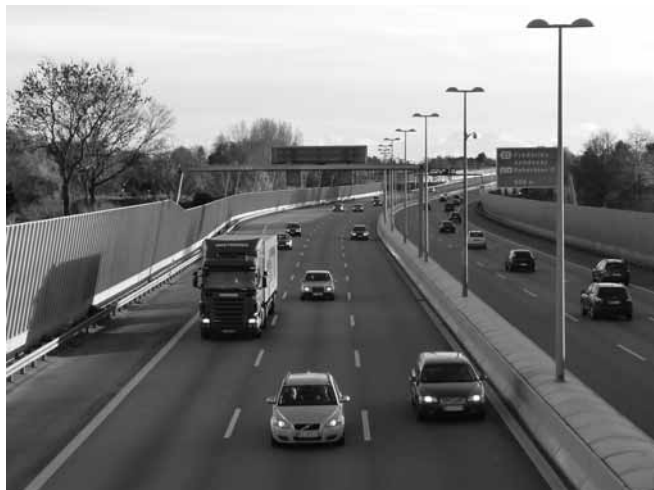
Figure 2. The M3 highway once completed, with porous asphalt and tilted 3m and 4m noise barriers.
